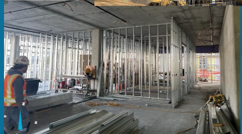
Building E Level 4 Interior Framing
